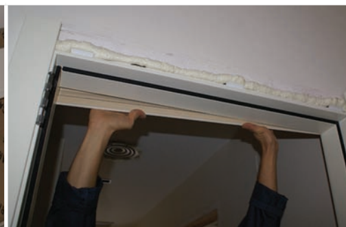
Colocar tapetas. Place architraves. Placer cafeutrement.
